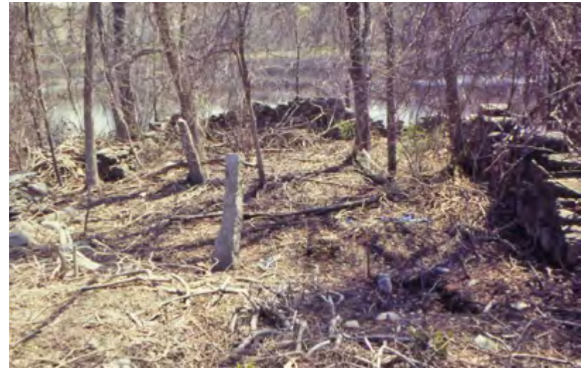
The granite piers seen here once supported the floor of the great barn, where travelers' horses were stabled.
