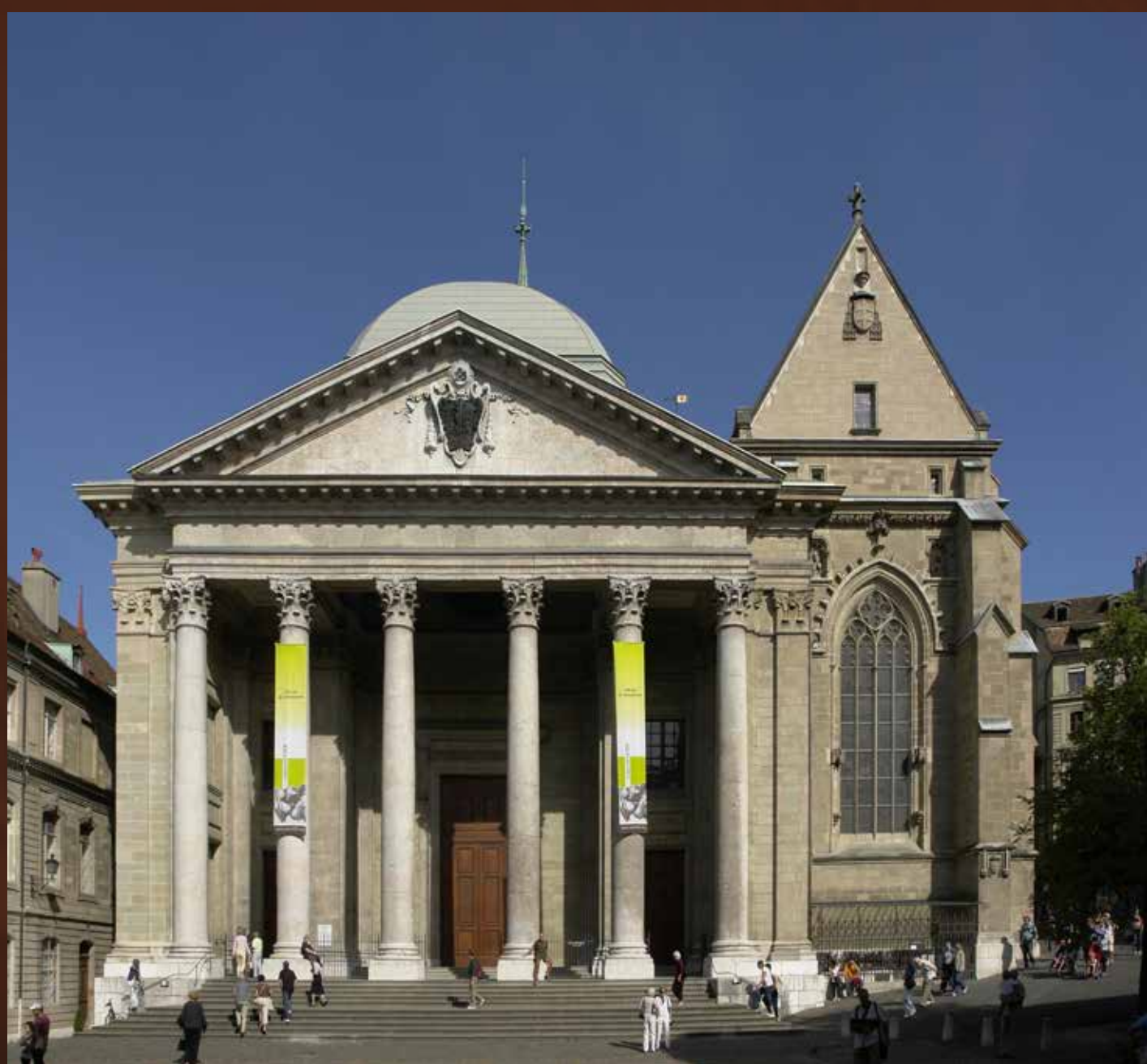
The former Catholic cathedral of St. Pierre in Geneva was the church mostly associated with John Calvin. YANN FORGET
