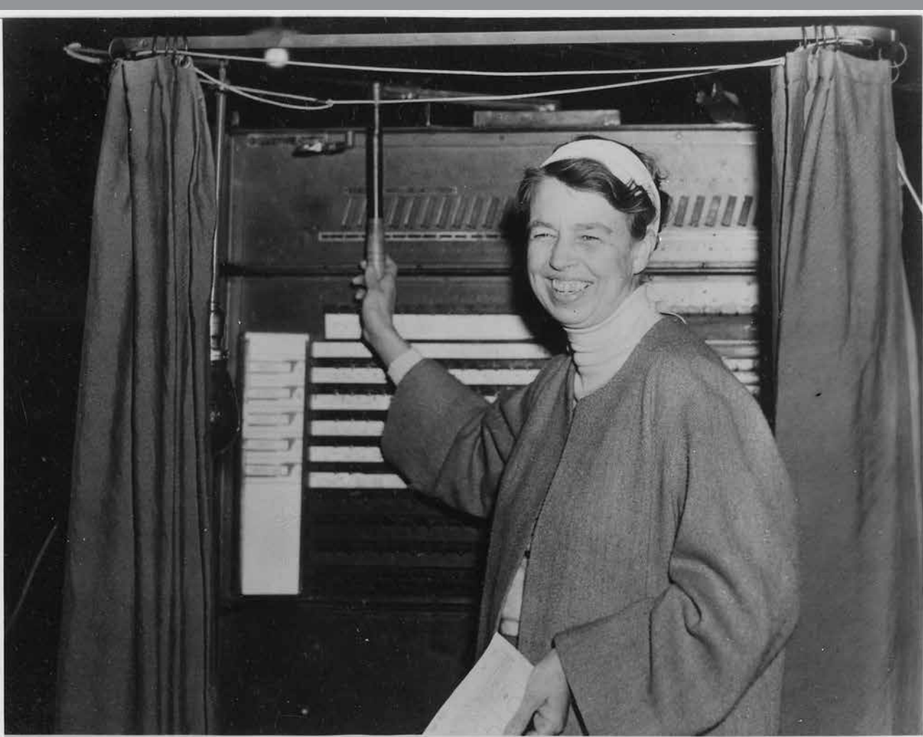
The voting machine used by Eleanor Roosevelt was mechanical, not electric. While there was no controversy, a broken “tooth” on a gear inside the machine could produce an inaccurate count. FDR LIBRARY PHOTO, NATIONAL PARK SERVICE
